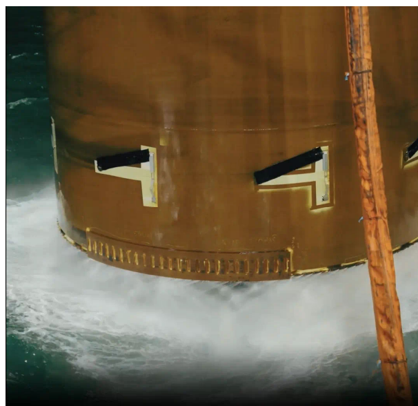
Figure 28. Field tests of pile with water jetting at the Gode Wind 3 wind farm (Ørsted).
