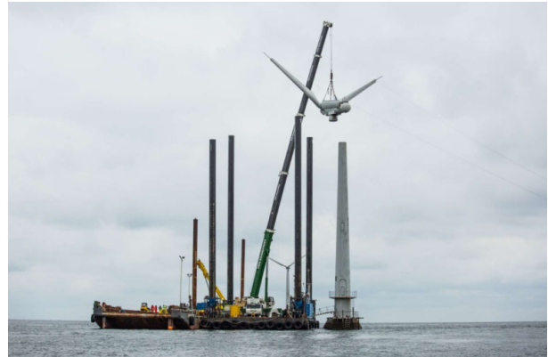
Figure 32. Decommissioning of the Vindeby offshore wind farm (source: Ørsted).
