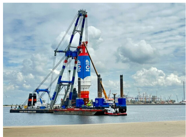
Figure 27. EQ-Piling technique (IQIP).
