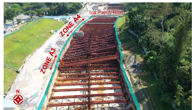
Figure 2. Aerial photograph of Zone A3 and Zone A4.
