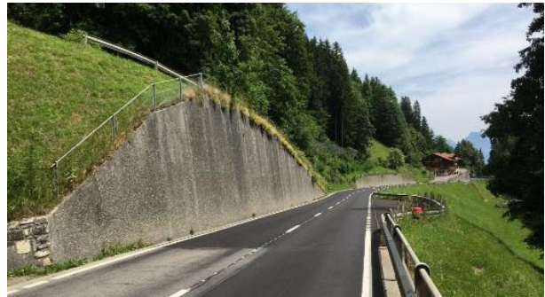
Figure 8. A good example of a crest line that follows the terrain harmoniously (Canton of Bern, 2023)
