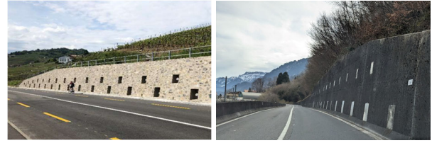
Figure 11. On the left, the recesses obscure the anchor heads, but the shadow creates contrast; on the right, the metal covers make the wall uniform. Pictures: canton of Vaud, PPIC.
