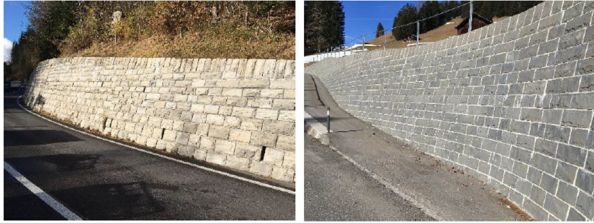
Figure 10. Good examples of layered natural-stone walls (Canton of Bern, 2023).
