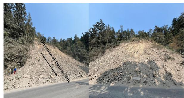
Figure 2. Failed slope with the direction of debris slope failure.
