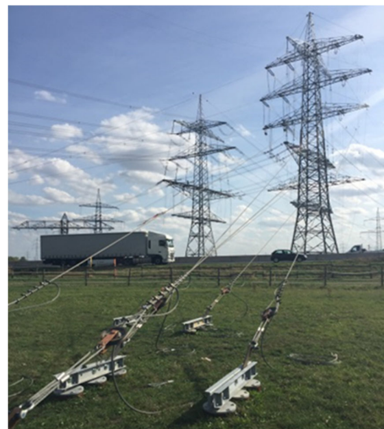
Figure 8. Anchoring with Spinnankers for a new 380 kV high-voltage line in Germany.
