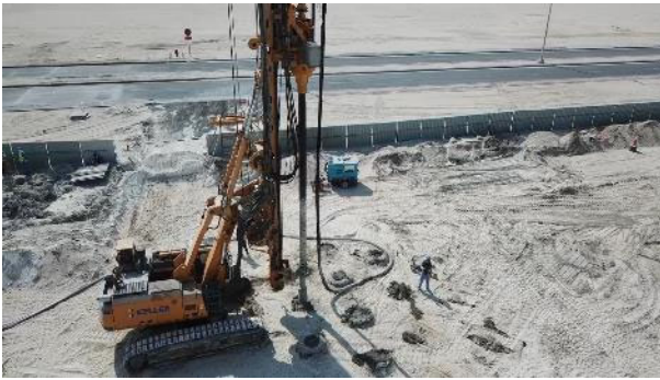
Figure 9: Installation of rigid inclusions
