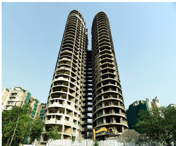
Figure 1. The twin towers located in the urban setting, pre-weakened and prepared for blasting.
