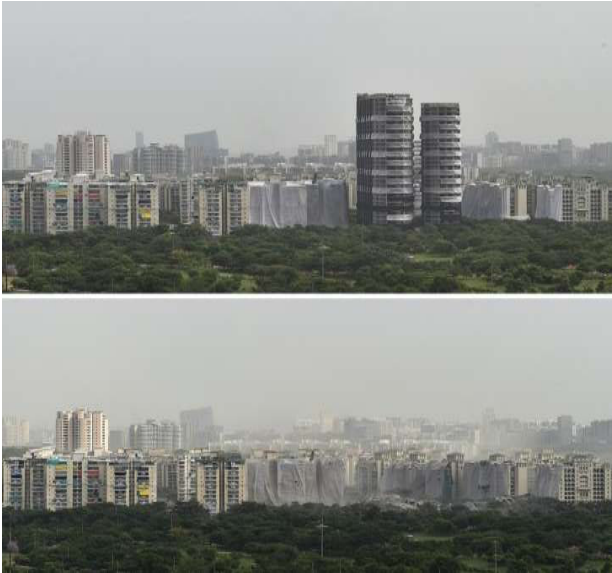
Figure 10. Pre- and post-demolition views of the Supertech Twin Towers, demonstrating successful collapse without damage to nearby infrastructure.
