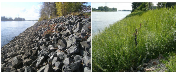
Figure 1. Riprap (left) and technical-biological bank protection measure with willow brush mattresses (right).
