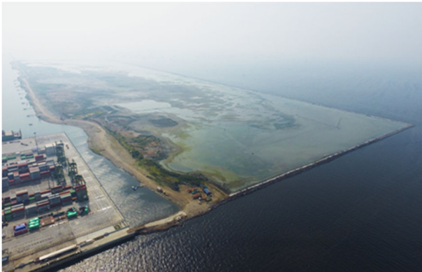
Figure 1. Slurry pond area at Kalibaru, Jakarta.
