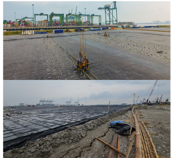
Figure 10. Implementation of the 1 st stage of ground improvement.
