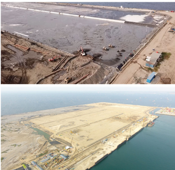
Figure 13. Hydraulic filling for embankment and surcharge preloading.
