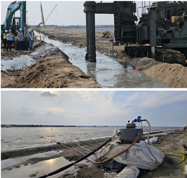
Figure 12. Implementation of the second-stage vacuum preloading.
