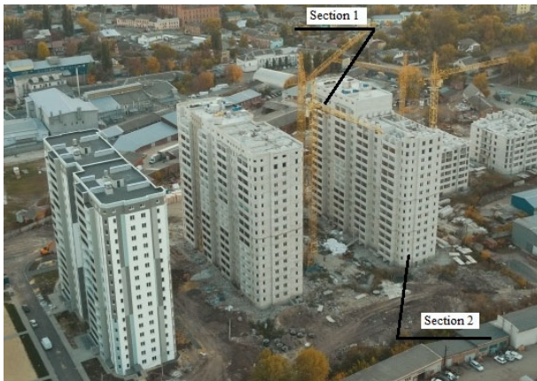
Figure 3. Location of Building 7 (Sections 1 and 2) under study during construction.
