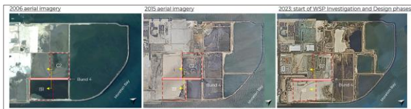
Figure 4. Aerial overview of land reclamation at PoB
