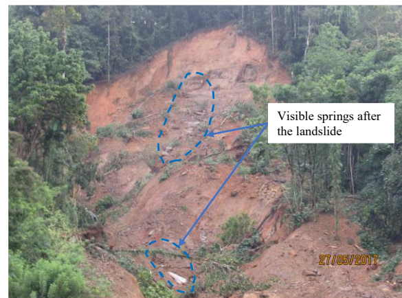
Figure 4. Springs emerge after the landslide
