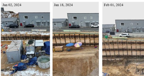
Figure 3. Excavation process of temporary earth retaining wall at Icheon site.
