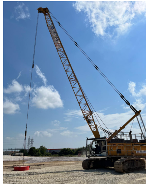
Figure 7. Ironing After Gravel Filling
