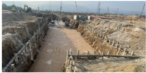
Figure 17. Shoring System with Jet Grout Columns and Steel Tubes
