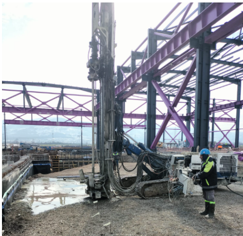
Figure 12. Jet Grout Application
