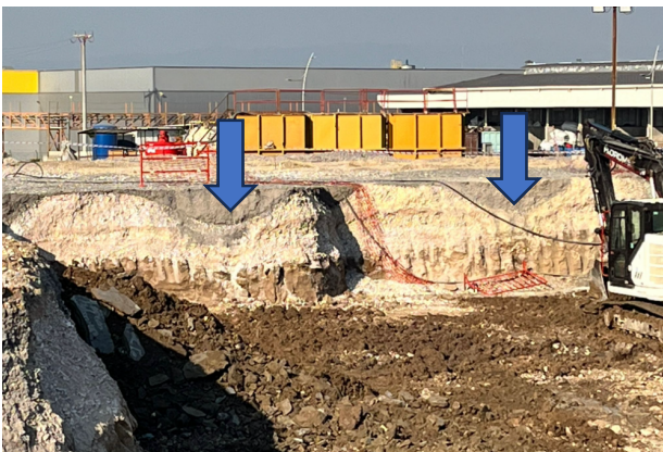
Figure 9. Densified Layers Observed in Excavation After Dynamic Compaction
