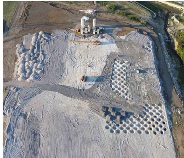
Figure 4. Dynamic Compaction - Site Photo
