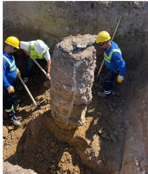
Figure 13. Diameter Measurements of Jet Grout Columns
