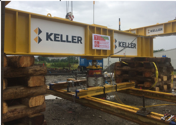
Figure 13. Pile load test arrangement
