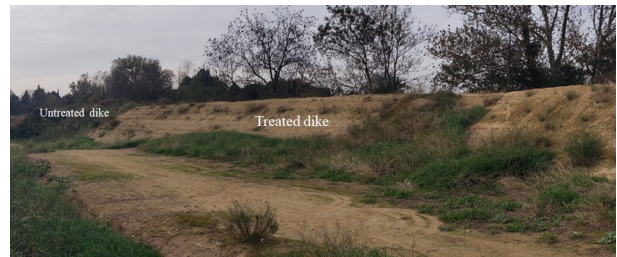
Figure 1. View of the dike built along the Vidourle river.
