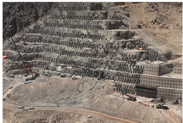
Figure 1. Construction progress photograph of the slope.
