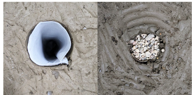
Figure 1. Sewn encasement placed in the hole with aggregate poured inside
