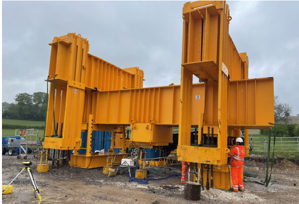
Figure 1. Reaction frame for the top loaded test pile at WDV.
