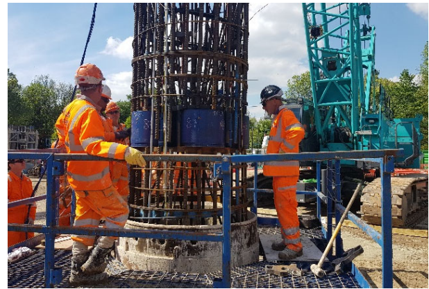
Figure 2. Photo at CVV test site.
