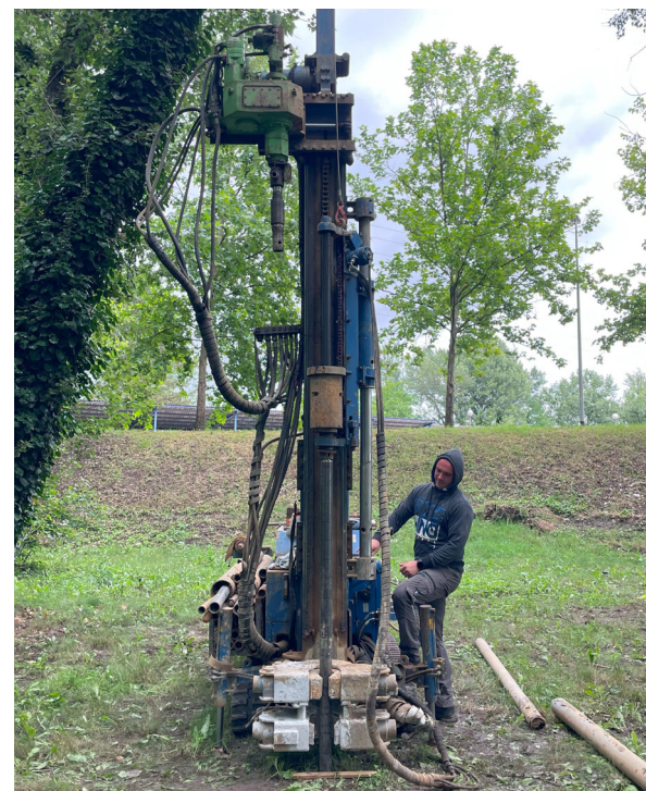
Figure 3. Collection of DPT data at Site 1 – University Hospital.
