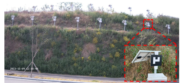
Figure 5. Field application of smart monitoring system at a steep slope site.
