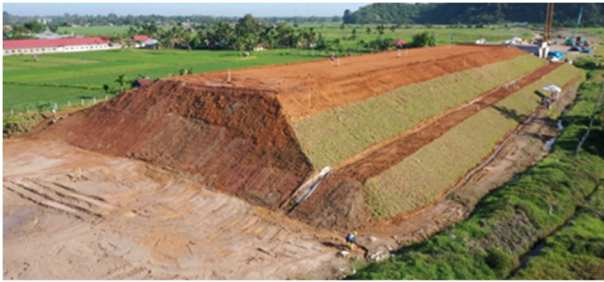
Figure 10. The maximum height of trial embankment (Himawan et al., 2024).
