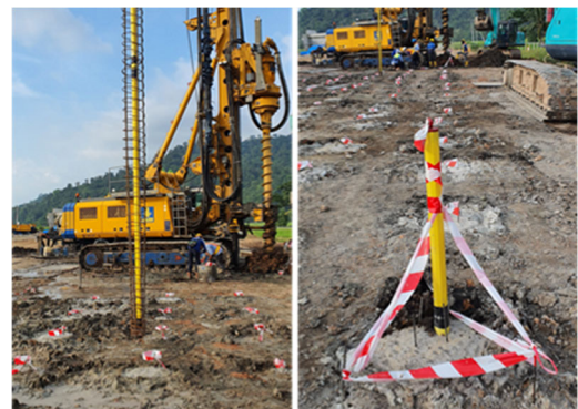
Figure 7. Inclinometer installation (Himawan et al., 2024).
