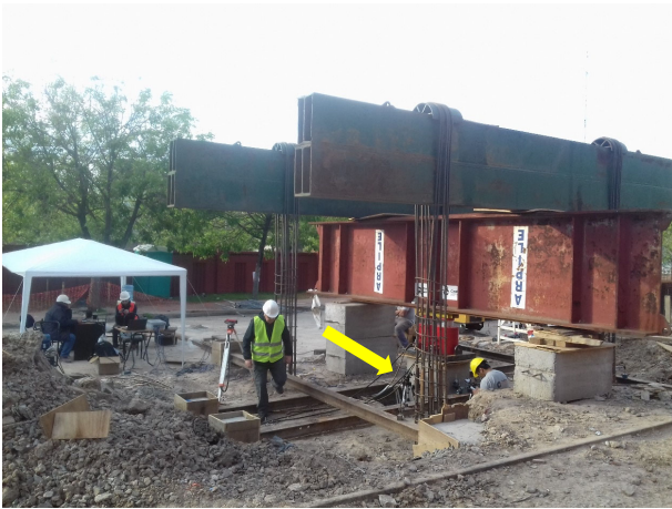
Figure 4: Execution of the drilled shaft axial load testing.
