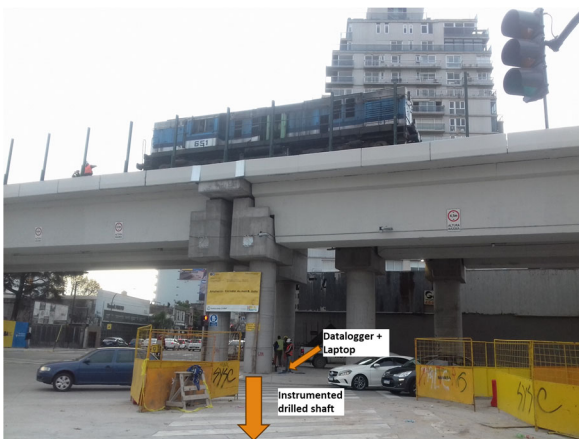
Figure 8: Strain measurements during viaduct deck load testing.
