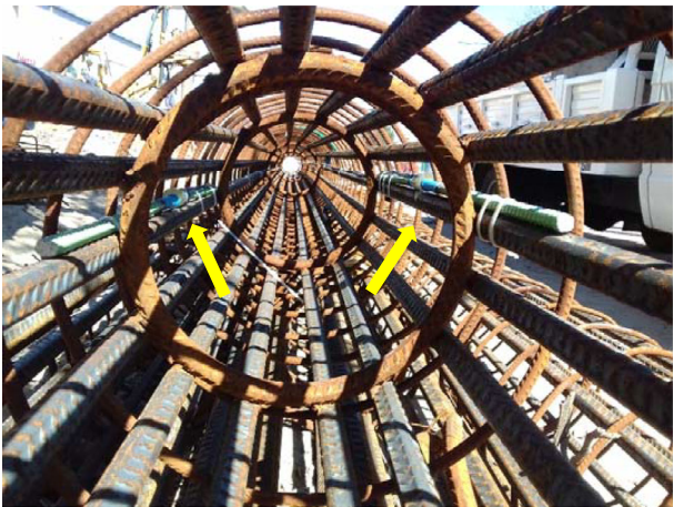
Figure 5: Strain gauges (sister bars) installed in the rebar cage.
