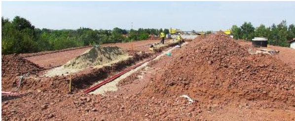
Figure 6. Installation of 3DSensor and reference inclinometer system.
