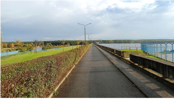
Figure 15. The earth dam equipped with DFOS sensors for distributed temperature (DTS) and acoustic sensing (DAS).
