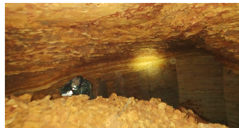
Figure 3. Fragment of a mine cavity affected by roof collapse.
