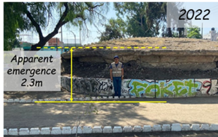
Figure 3. Shaft 7, Eastern Interceptor (Eduardo Molina).
