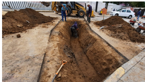
b) Excavation for strain dissipation trench.
