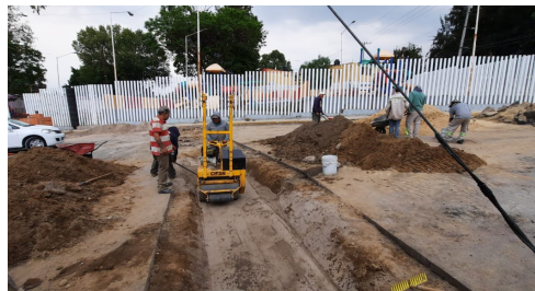
c) Placement of granular material fill and compaction.
