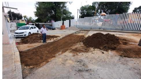
d) Preparation of pavement base for placement of asphalt.
