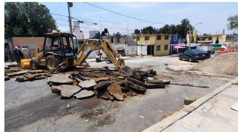
a) Cutting of asphalt pavement on road.
