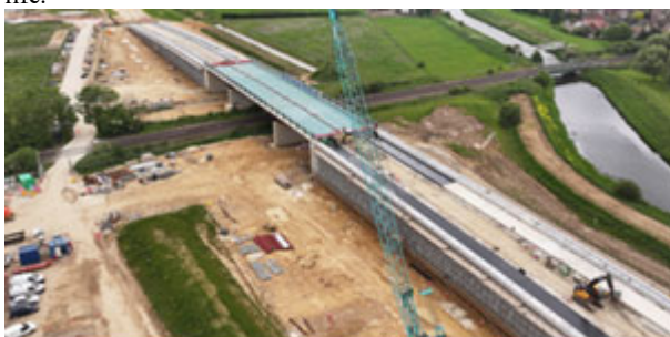
Figure 1. LWA Fill and HDPE Geogrid
