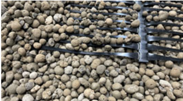
Figure 2. LWA Fill and HDPE Geogrid
