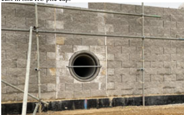
Figure 8. Badger tunnel construction
