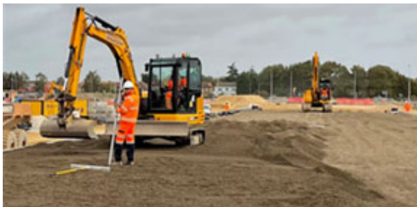
Figure 8. Placement of LWA fill using tracked plant
