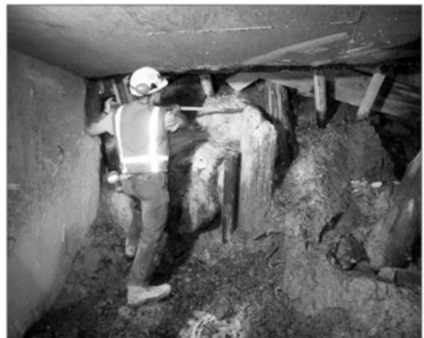
Figure 34. Removal of timber piles and other obstructions, after Powderham and O'Brien 2020.
