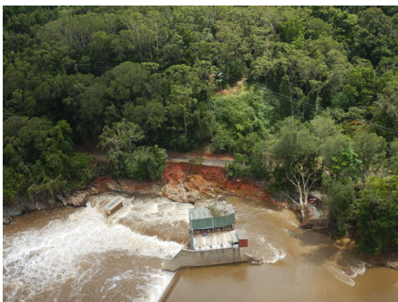
Figure 2. Aerial photo of the affected site (taken from a helicopter).
