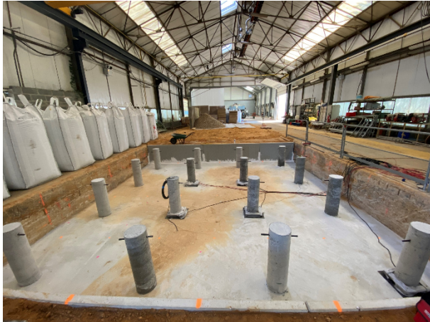
Figure 1. Experimental pit, Cerema.
