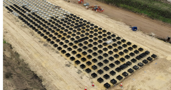
Figure 9. Finished pile layout (pile caps visible, 2.5m spacing)
