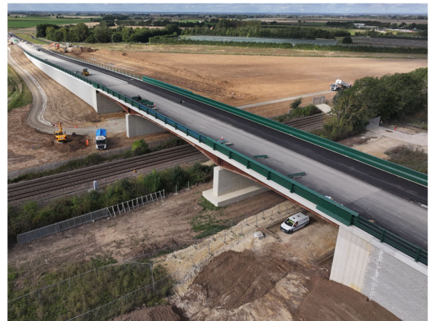
Figure 4. Railway bridge in construction
