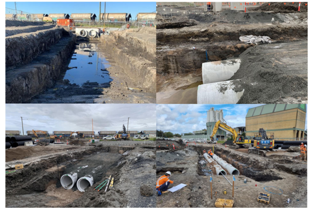
Figure 14. MSM block after excavation and during pipe installation.
