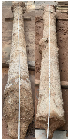
Figure 8. Exhumed piles post jet washing: bentonite (left) and polymer (right)
