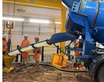
Figure 3. Placement of concrete in the bore via the tremie method
