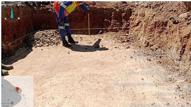
Figure 3. The excavated area of the A56
