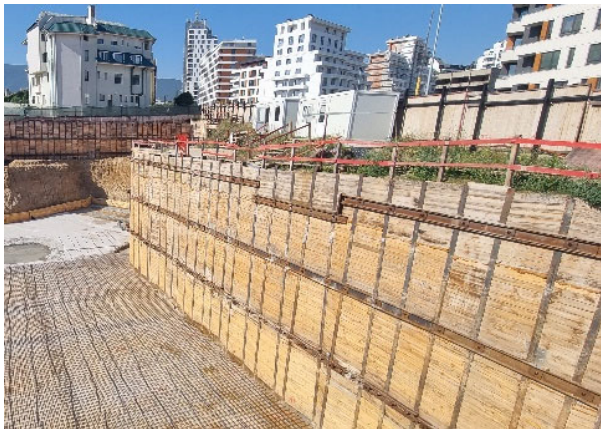
Figure 1. A retaining wall
