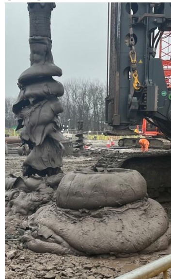
Figure 4. Alluvial arisings from rotary bored piling rig.
