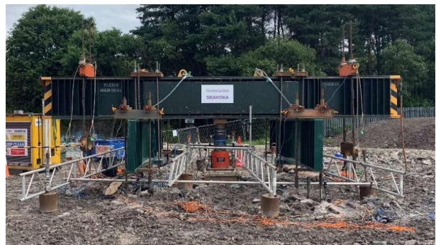
Figure 8. Sacrificial test pile setup with 6no. anchor piles.
