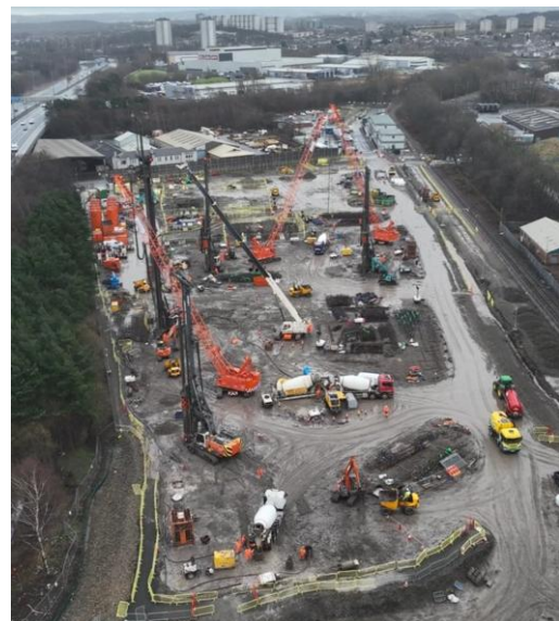
Figure 1. SCEC construction site during piling operations.
