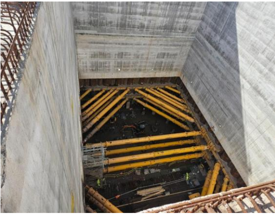
Figure 7. Combi-wall installation & temporary propping.
