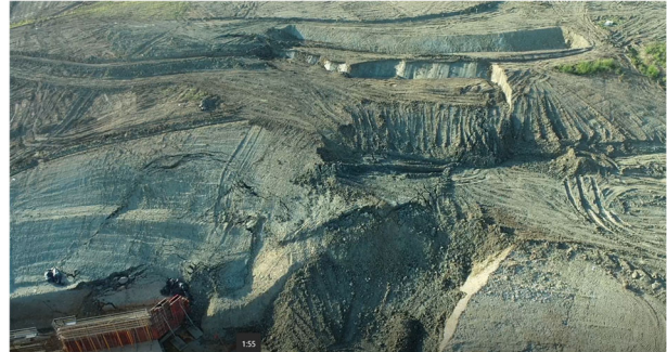
Figure 4. Slope stability problems arising on a clayey mine spoil heap.
