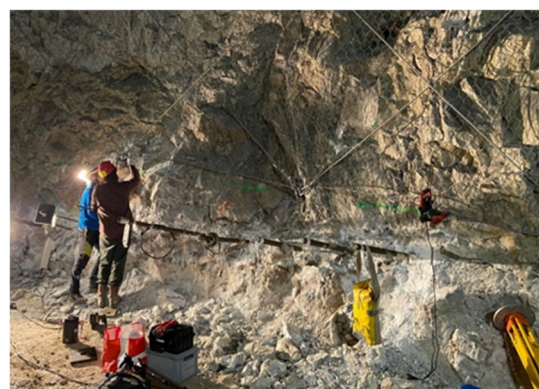
Figure 3. Wall with anchors in Santa Brigida cave.
