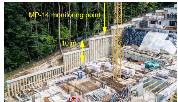
Figure 5. Final construction stage.
