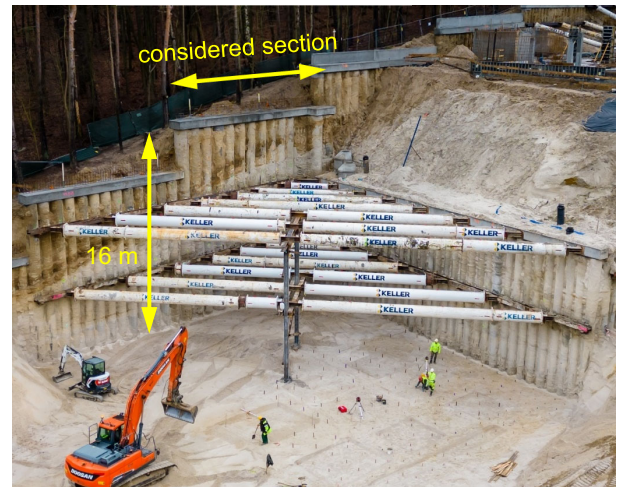
Figure 4. Temporary construction stage.
