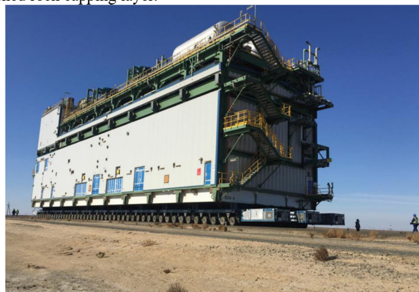
Figure 3. Typical module transport of a pipe rack
