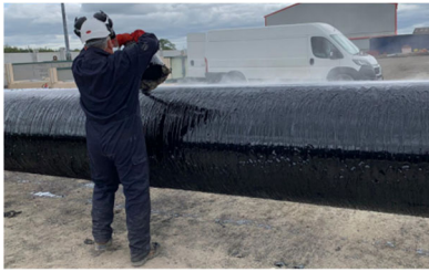
Figure 5. Bitumen coating application on permanent casing
