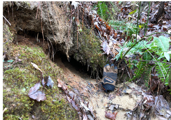
Figure 1. Photograph of the soil pipe outlet at a landslide site in West Alabama. The eroded sand can be seen below the glove at the pipe outlet.
