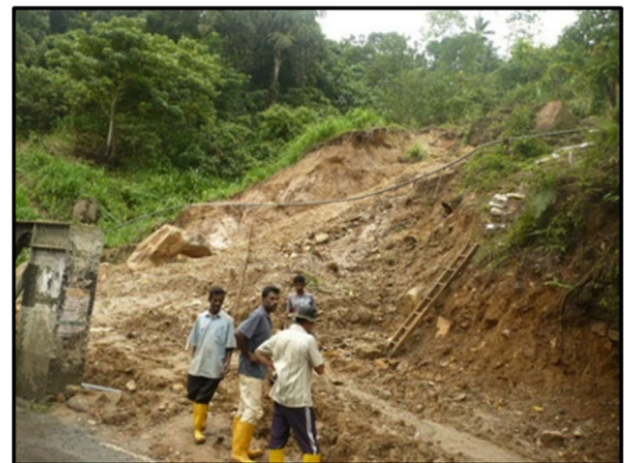
Figure 2. Photograph just after the failure
