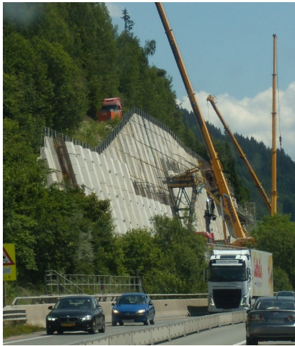
Figure 2. Egger wall at the A10 highway during its strengthening.
