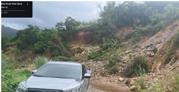
Figure 3. Example of a landslide on East-West Road after heavy rainfall (image source: Google Maps, accessed June 2025).
