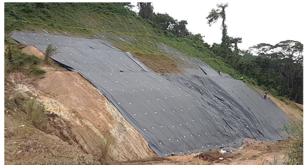
Figure 5. Renovated embankment in Nasugbu.
