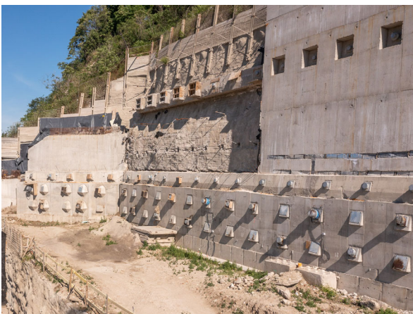
Figure 6. Concrete beams with wall in the upper part of slope.
