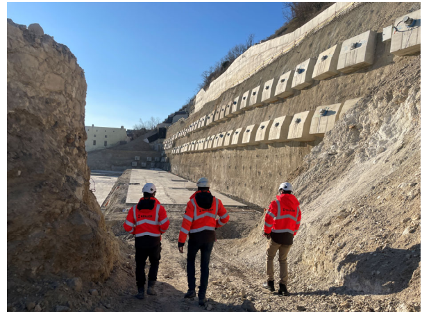
Figure 7. Concrete plinths in the lower part of the stabilization.
