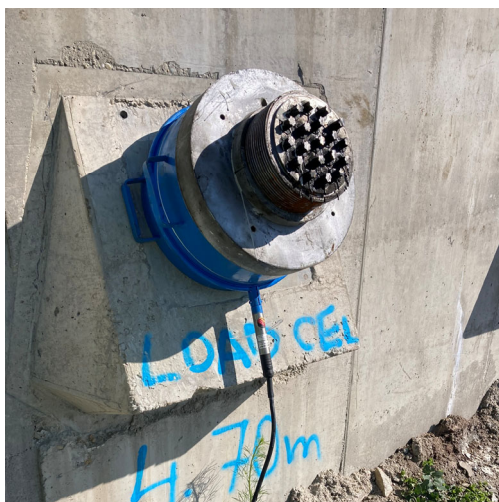
Figure 8. Anchor with dynamometer (photo before final coverage).
