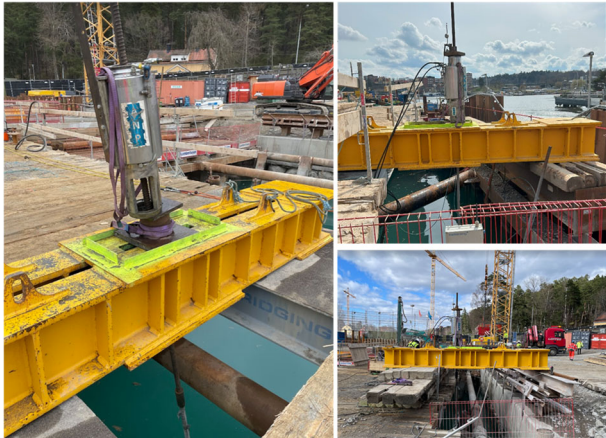
Figure 11. Testing permanent anchors against a temporary bridge.
