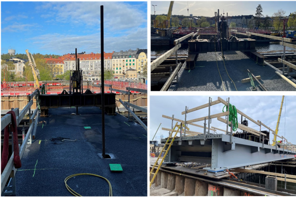
Figure 6. Testing uplift piles against a temporary bridge.
