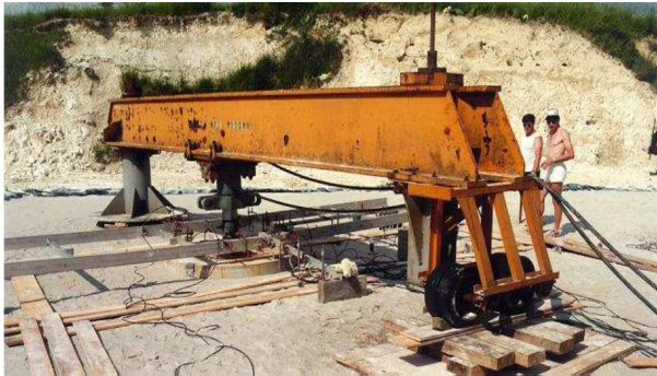
Figure 1: Foundation loading tests on Labenne performed by LCP
