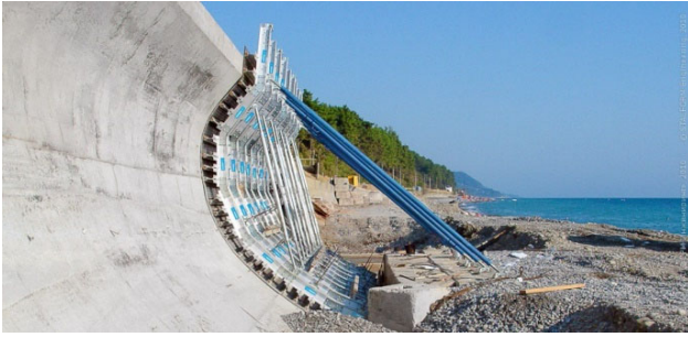
Figure 2. Sea breakwater wall of shore protection in Yalta
